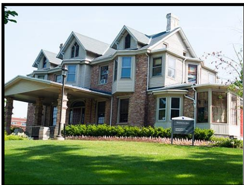
Wiestling Hall, Built in 1807 as Hughes Mansion
